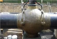
Kebu Petro-Tape A303 is a cold-applied corrosion protection tape. When applied in three layers the Kebu Petro-Tape A303 meets the requirements of DIN EN 12068 and DIN 30672, load class A at a maximum operating temperature of 30 °C.
