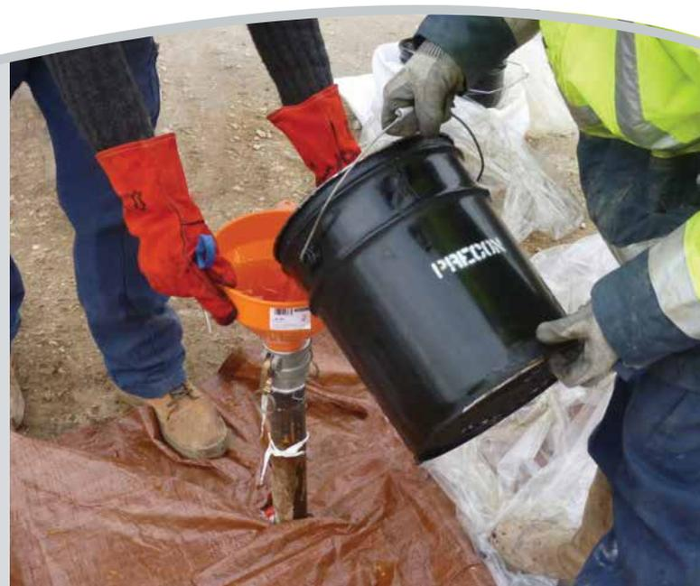
*Trenton Pre-Con™ mitigates any corrosion that would be caused by water left in the casing.*
